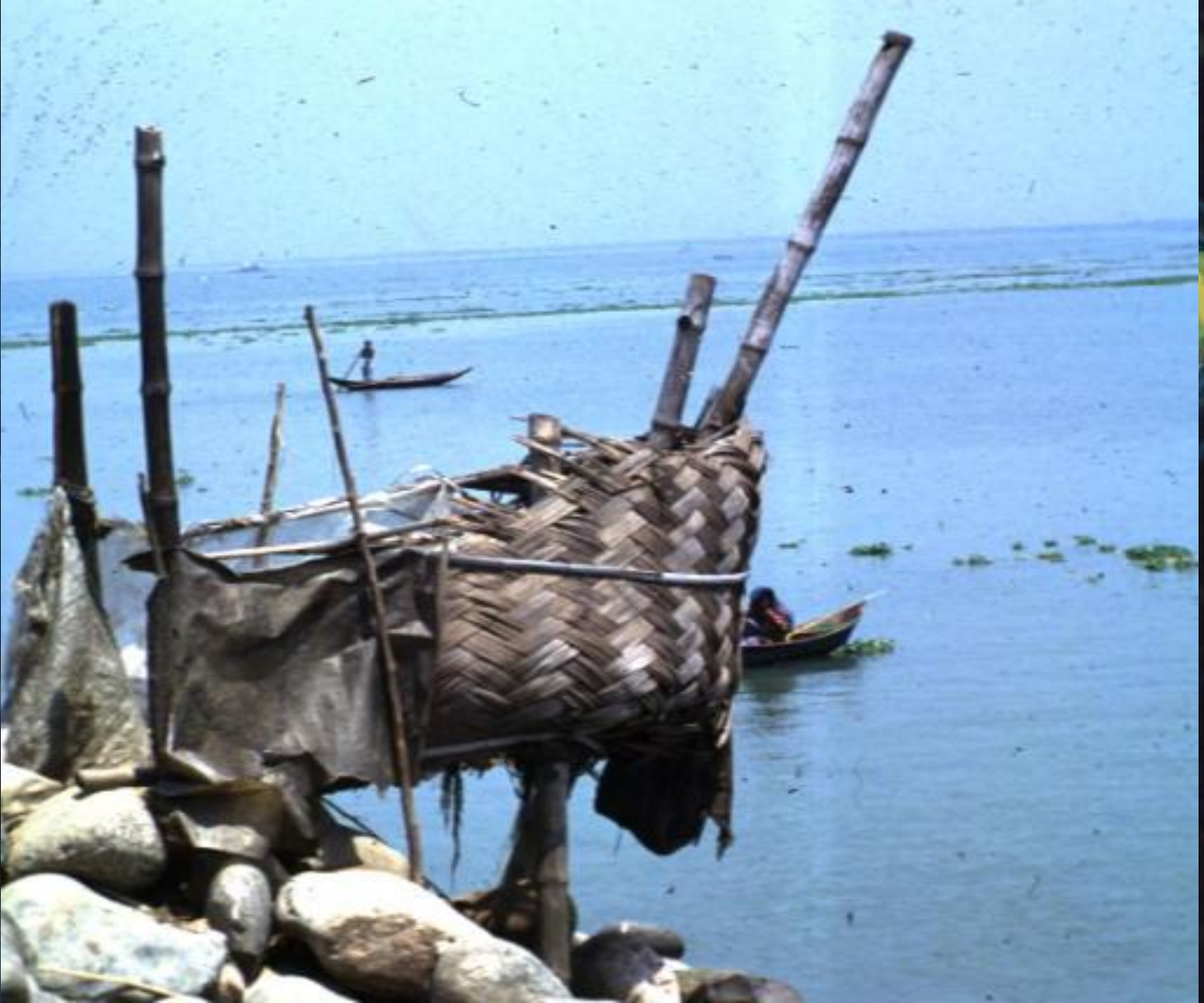
■ Hanging latrine on Meghna River, Nepal
