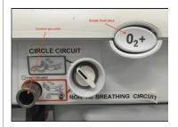
When pressed, oxygen bypasses the back bar and is delivered to the CGO (common gas outlet) at >35 L/min.
